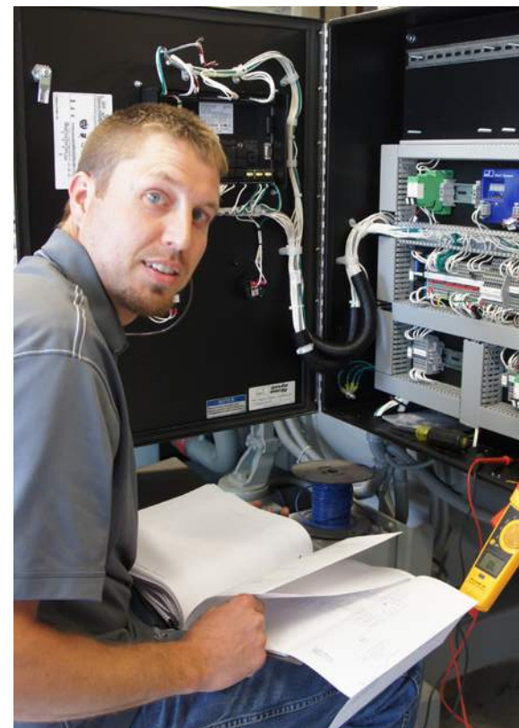
KEVIN WORKING ON A GENERATOR
